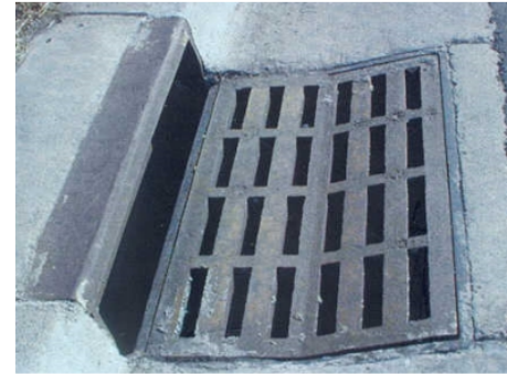
Figure 2-4 Combination Drain Inlet ("Drainage Design" 16).
